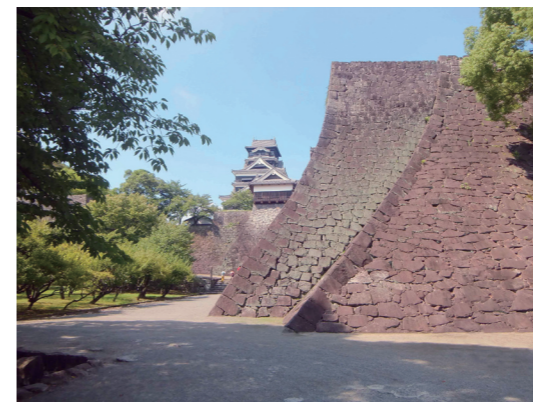
The two stone walls below the main enclosure of Kumamoto Castle. (Right, the Katō-era wall; left, the Hosokawa-era wall.) 熊本城本丸下の二重の石垣(右が加藤時代、左が細川時代)
